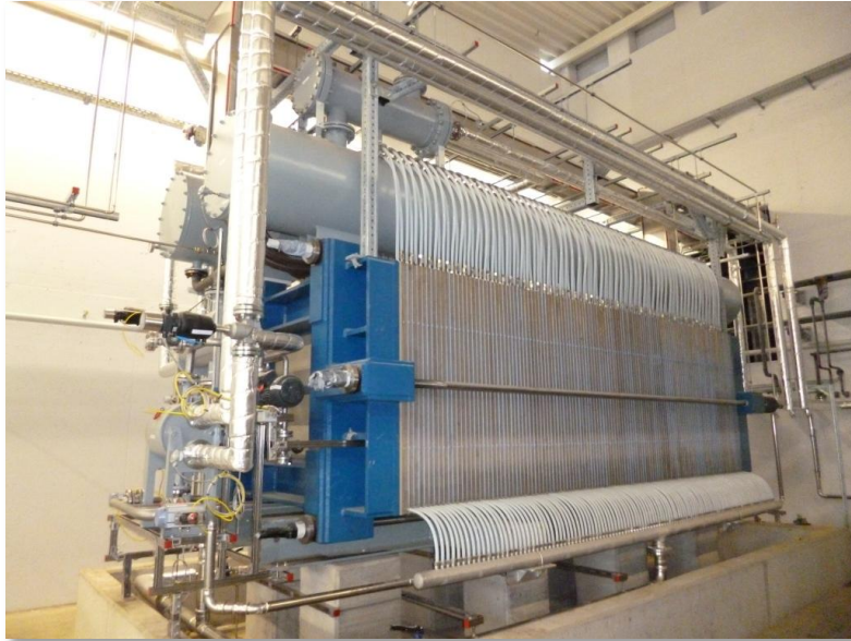
Electrolyser (3 x 2 MW)
